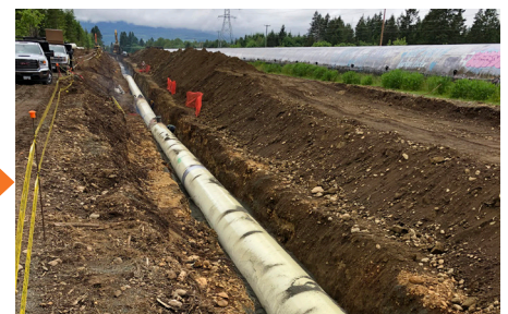
Pipe is installed in the trench. (May 2020)
