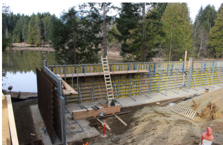
Formwork for the electrical building started earlier this year. (Mar. 2020)
